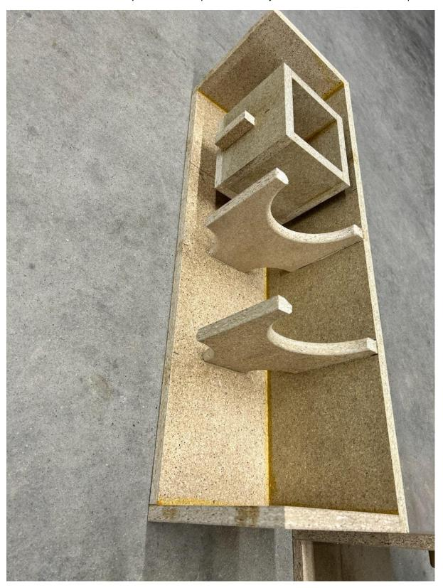
Materials of construction in this case was particle board shelving from Menards. It has become a popular option for cabinets that have all dimensions smaller than 11-1/4" or so. Total cost for these cabinets in unfinished state is less than \$50! That makes this a true budget design.
